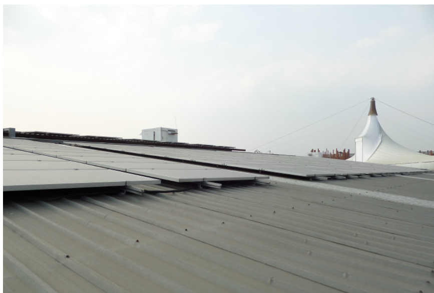
Solar Rooftop Installation at Porto Chino
